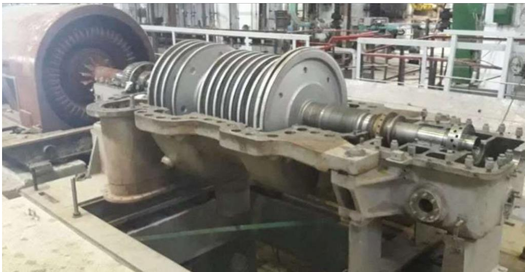
Slika 3. Remont parne turbine K-300-240 LMZ [5]
