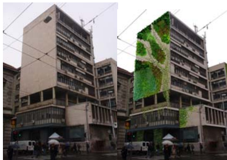
Fig. 3. Building before and after intervention
