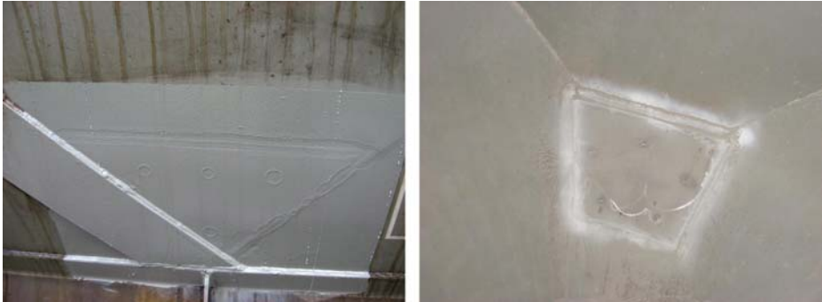
SI.6 Crack repair on the tanks
